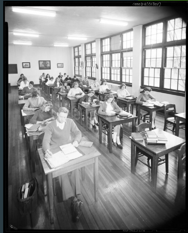
John Burroughs School, Classroom. 34-1301, Charles Trefts Photographs, SHSMO
